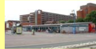
Extensions of Town Centre CCTV System – Waltham Cross Bus station
