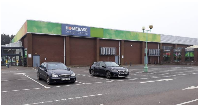
Figure 8 Existing Homebase Store (north elevation)
