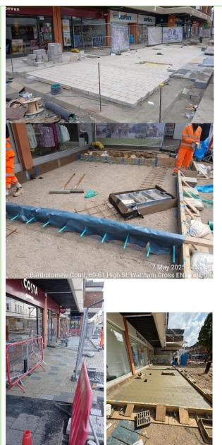
Drainage works (installation of gullies).
