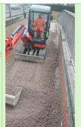
Park Lane to northern end of the High Street (adjacent to Wickes) Lowering of existing utility ducts to accommodate new road surface.
