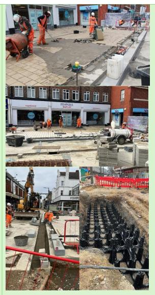
Park Lane to northern end of the High Street (adjacent to Wickes) Excavation for tree cell installation, backfilling of diverted electricity cable, excavation for kerb braces, parking bays and footpath concrete foundations.
