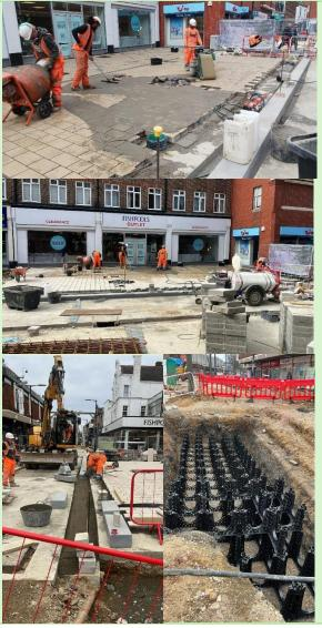
Excavation for tree cell installation, backfilling of diverted electricity cable, excavation for kerb braces, parking bays and footpath concrete foundations.
