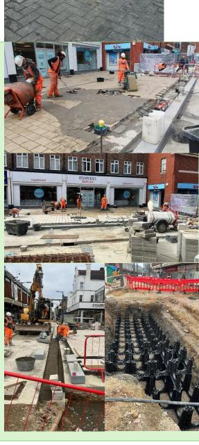
Excavation for tree cell installation, backfilling of diverted electricity cable, excavation for kerb braces, parking bays and footpath concrete foundations.
