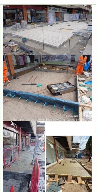
Drainage works (installation of gullies).
