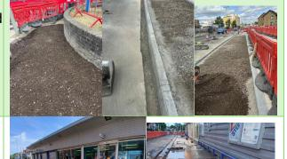
Excavation and preparation for concrete bays and concrete pouring at bus shelter.
