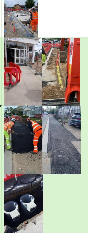
Installation of edgings, laying of paving and grouting in east wing market area and in front of Costa Coffee.
