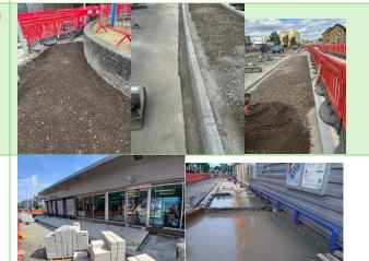
Excavation and preparation for concrete bays and concrete pouring at bus shelter.
