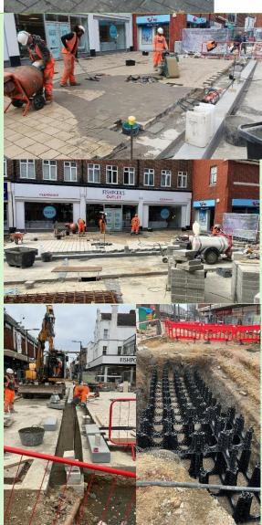
Excavation for tree cell installation, backfilling of diverted electricity cable, excavation for kerb braces, parking bays and footpath concrete foundations.
