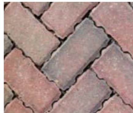
Permeable block paving
