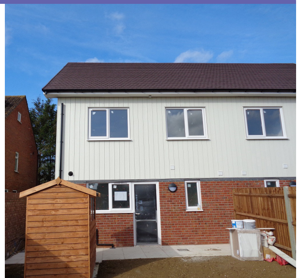
New affordable housing at Beltona Gardens, Cheshunt.
