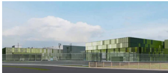
Google data centre
