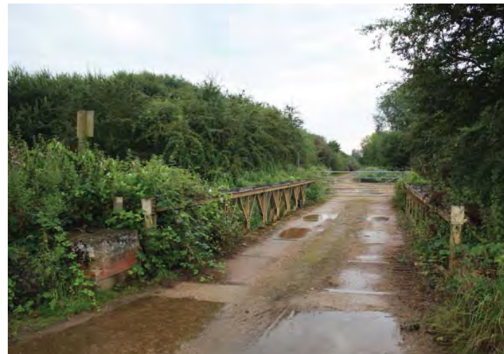
North entrance bridge and haul road beyond
