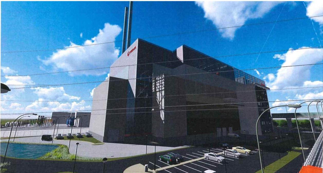
The contents of this structure would include a tipping hall, an incineration chamber, a boiler hall, various treatment facilities, an administration building and a visitor centre. The main building would be 48 metres in height (the adjacent Rye House Power Station is 28 metres). There will be two chimneys of 87 metres in height (the adjacent power station chimneys are 58 metres).
